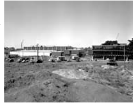
Building blocks (1962): The Hargrave Library (right) and Science buildings – Administration, Physics and Chemistry. Photo courtesy of Monash University Archives, Image 5040.
